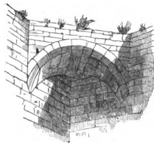
Squinch, Canon's Ashby, Northamptonshire.
