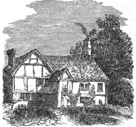
Milton's Cottage at Chalfont.
