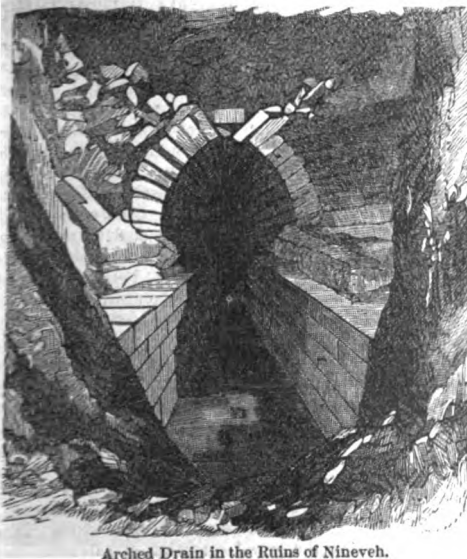
Arched Drain in the Ruins of Nineveh.
